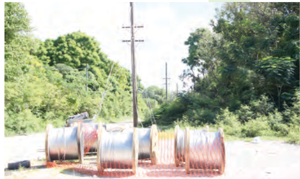
Solar Interconnector Overhead Line under Construction
