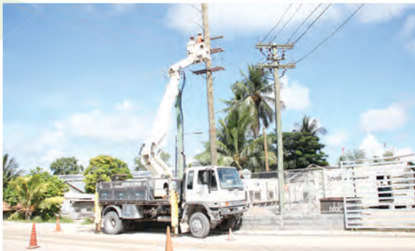
Solar Interconnector / Field Feeder under Construction
